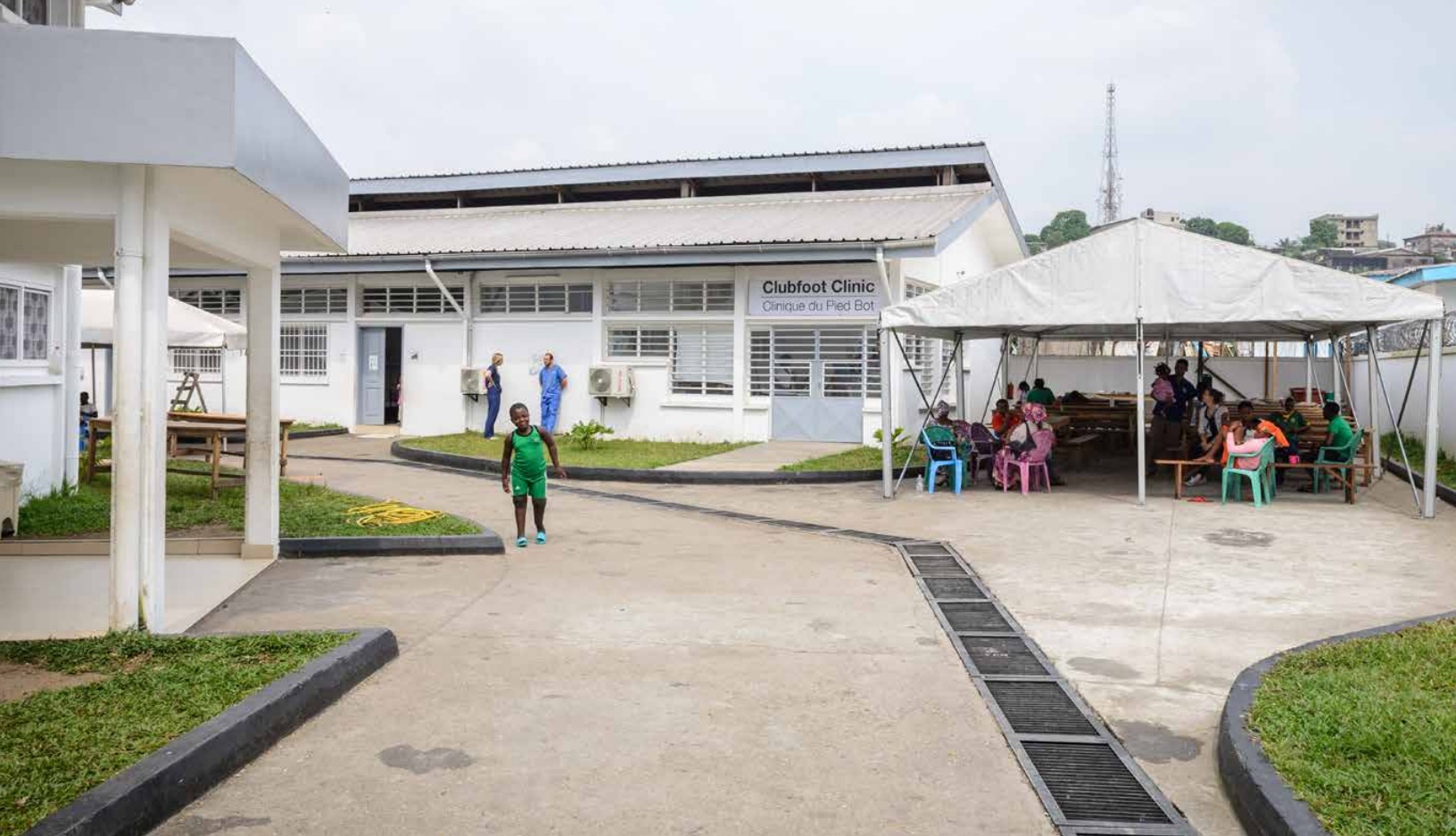
HOPE Center shortly after the renovations were completed – also the site for the Ponseti Clinic CMA171205_HOPE_CENTER_SL007
